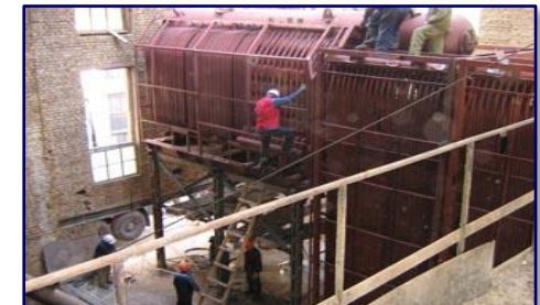
Installation of superheated steam boiler 15 MW
