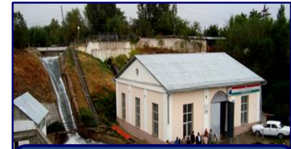
Two small hydro power units (2 x 500 kW)
